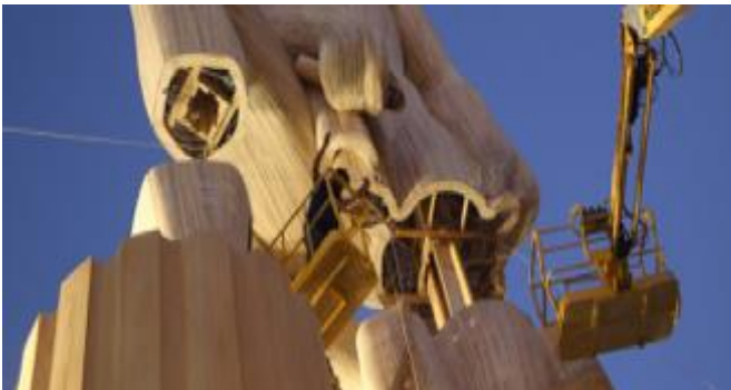
Picture 18 Image of "Fallas" construction
