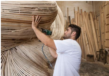
Picture 28 “Vareta” construction
