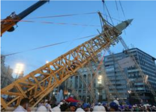
Picture 17 Image of "Fallas" construction
